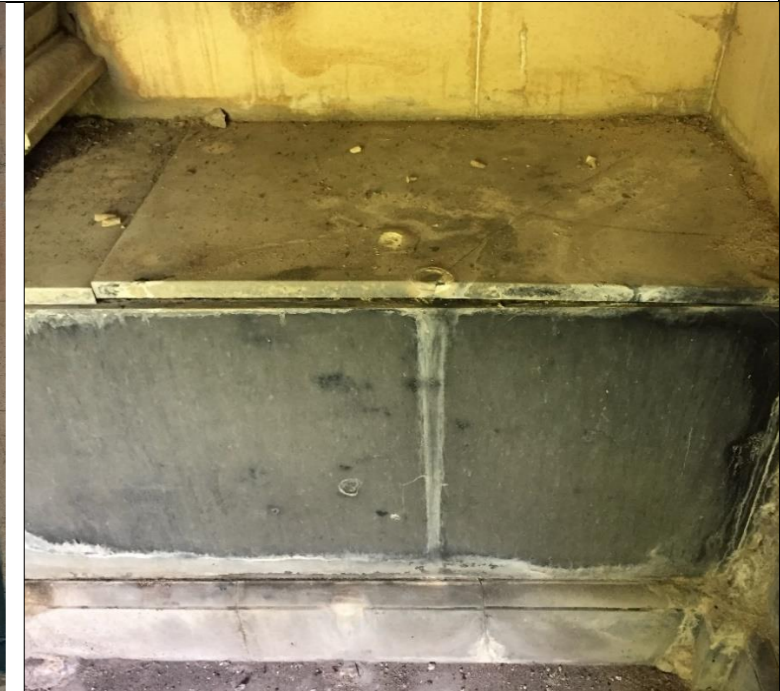
Lifted marble slab to plinth
