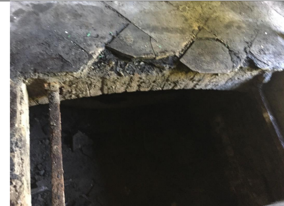
Brick arch of vaulted crypt beneath
