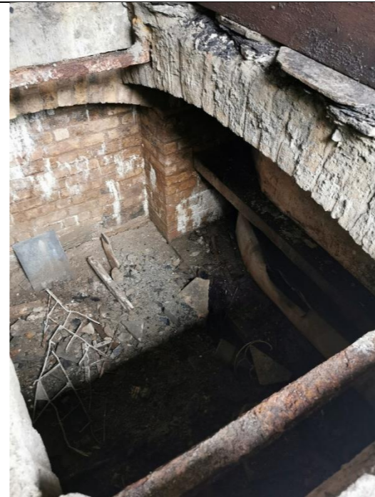
View of brick vaulting to crypt
