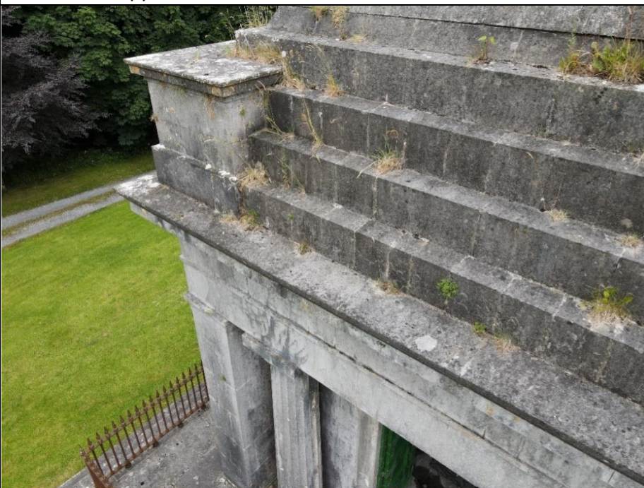
View of cornice and steps to base of pyramid
