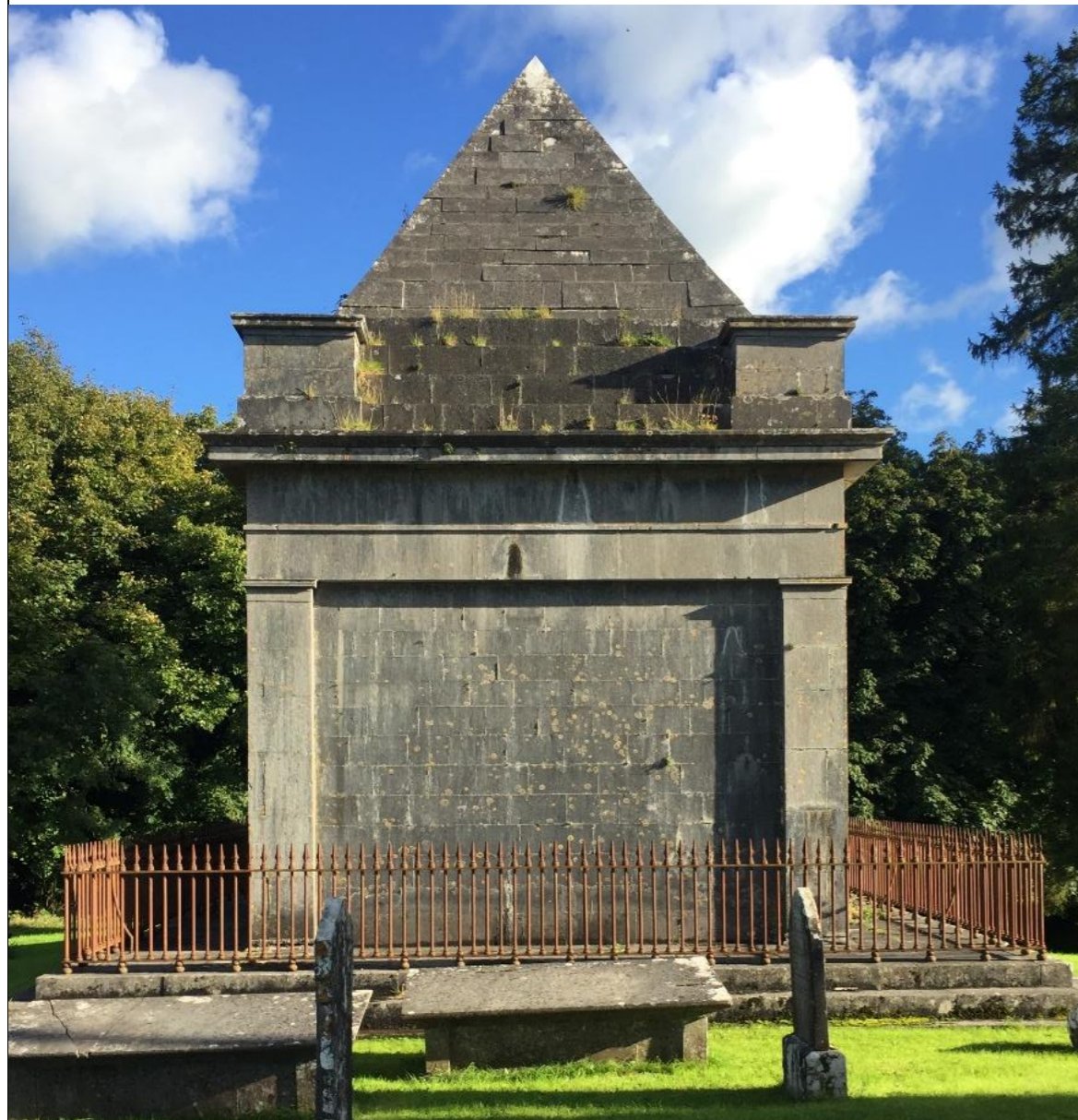
Water saturation to external cornice
