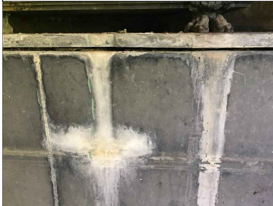
Calcite water staining
