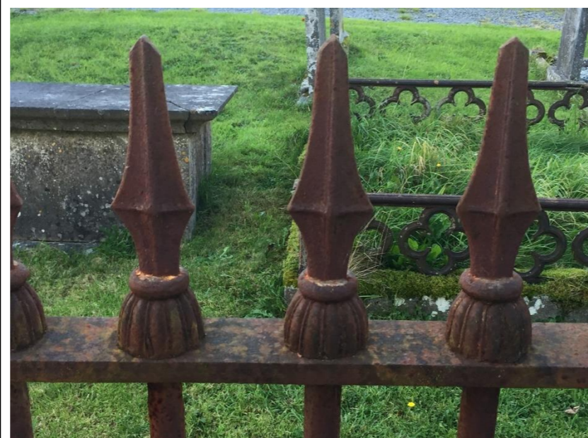
Wrought and cast-iron railing detail
