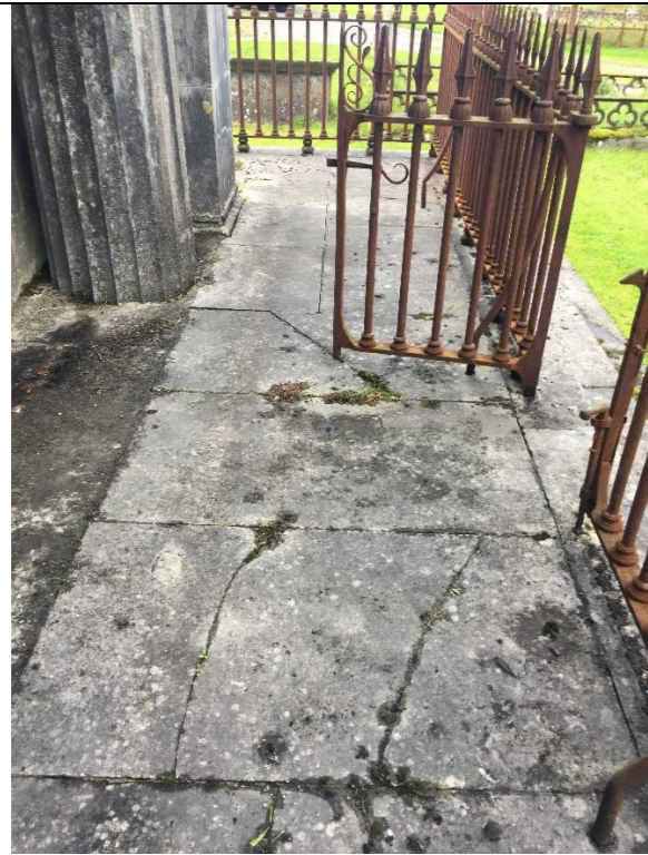
Stone paving inside entrance gates to north-east
