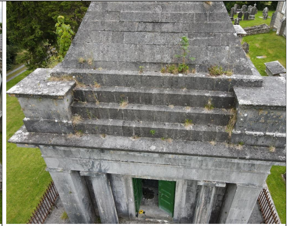
View of limestone cornice and stepped base to front
