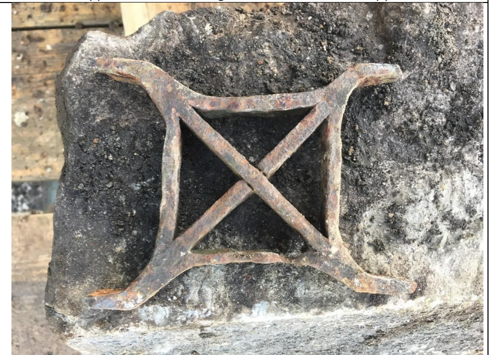
Wrought-iron vent detail
