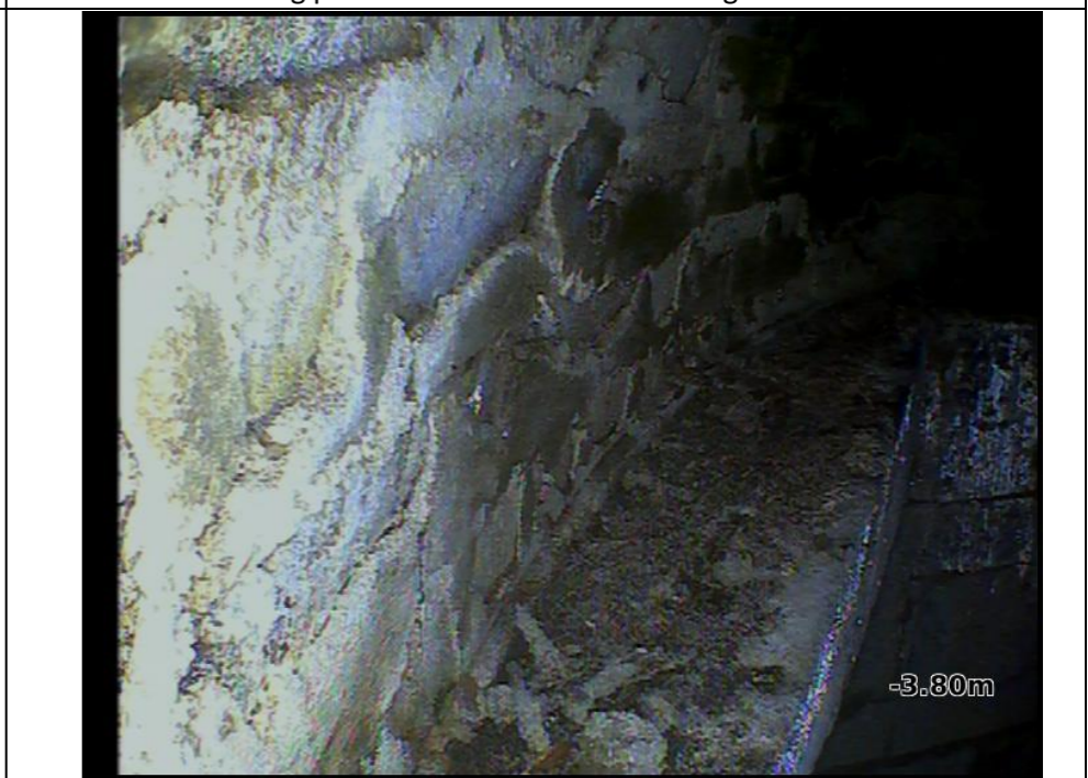
Stone ledging to perimeter of dome
