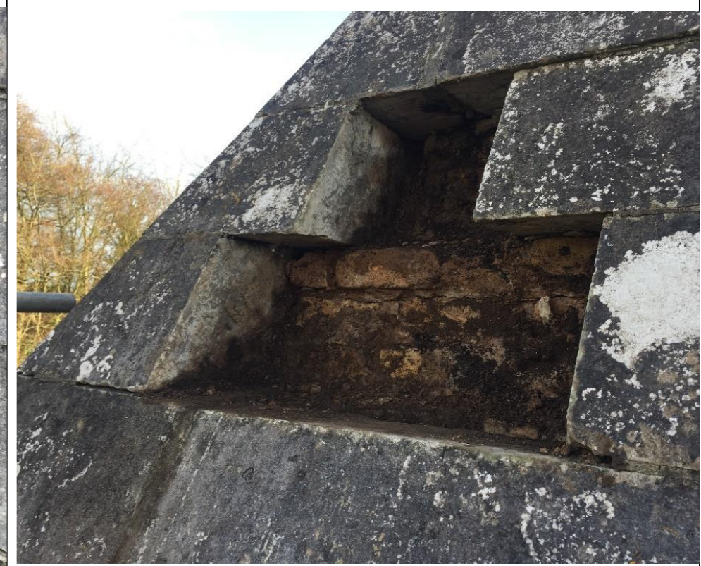
Stepped brick inner-lining behind ashlar limestone pyramid
