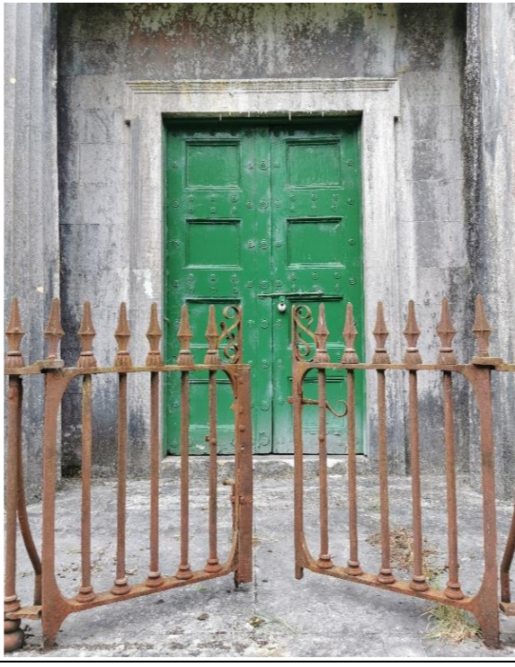
Entrance doorcase with cut stone surround
