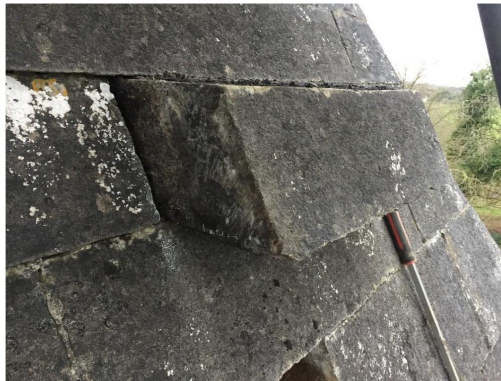
Limestone block being removed during opening-up works
