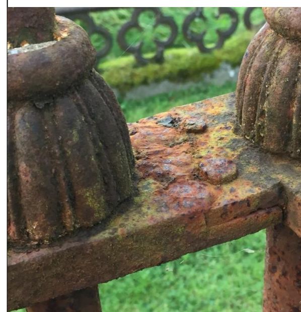
Pins and railing junctions
