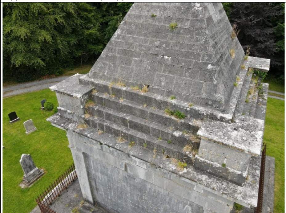
View of limestone cornice and stepped base
