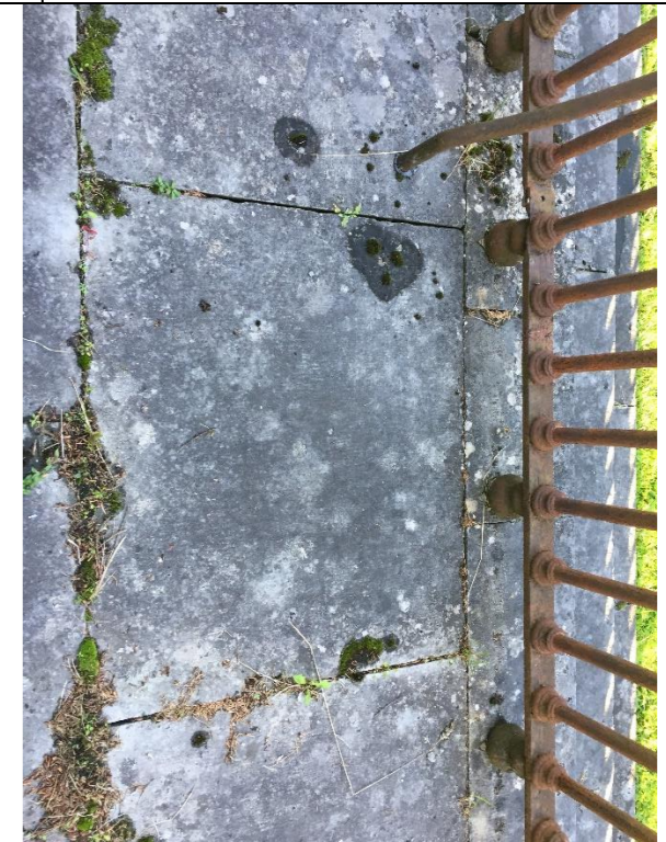
View of paving to south-east
