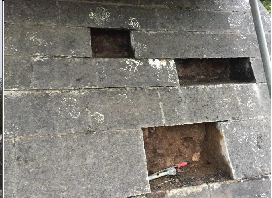
Stone blocks removed to lower pyramid during opening up works 2022
