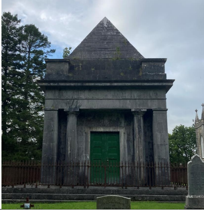
Front elevation of Malone mausoleum
