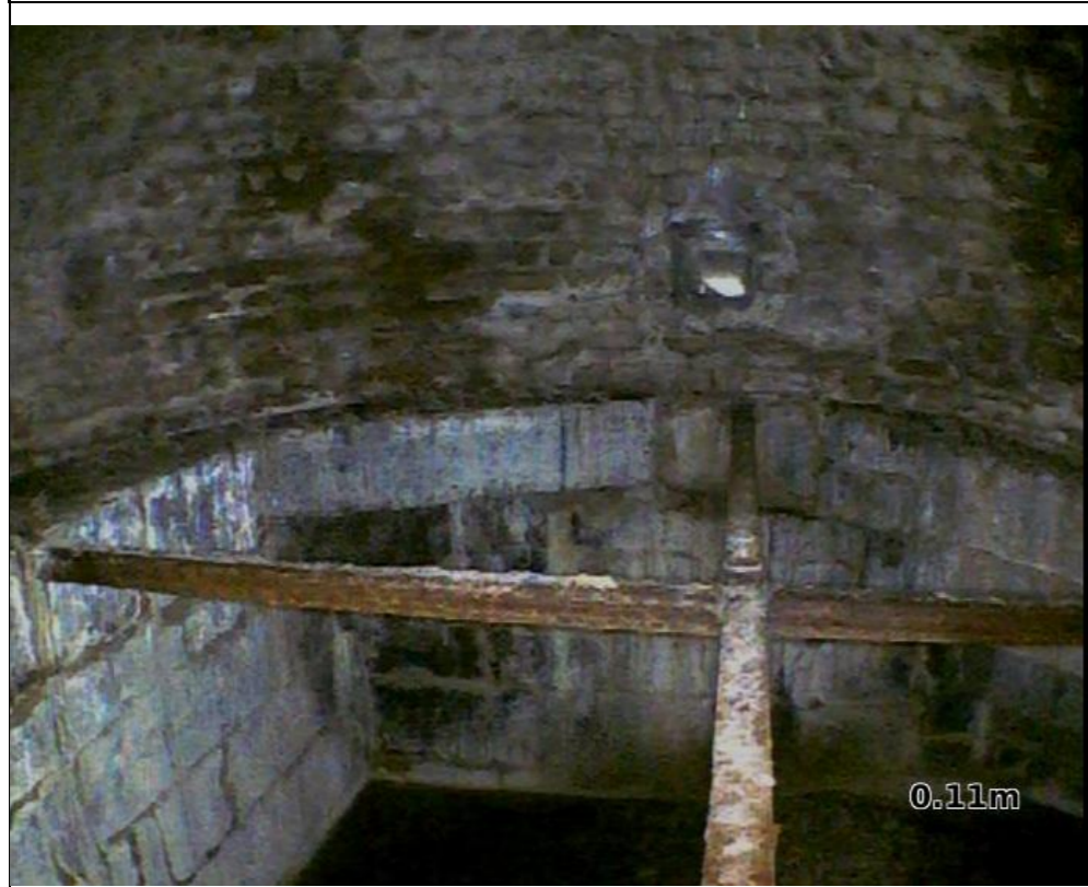
Wrought-iron bracing and view of lower limestone courses
