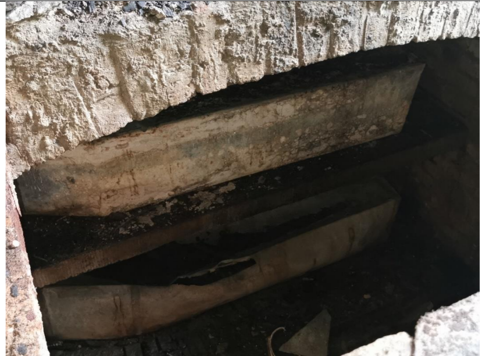
Lead lined caskets and limestone shelf within crypt
