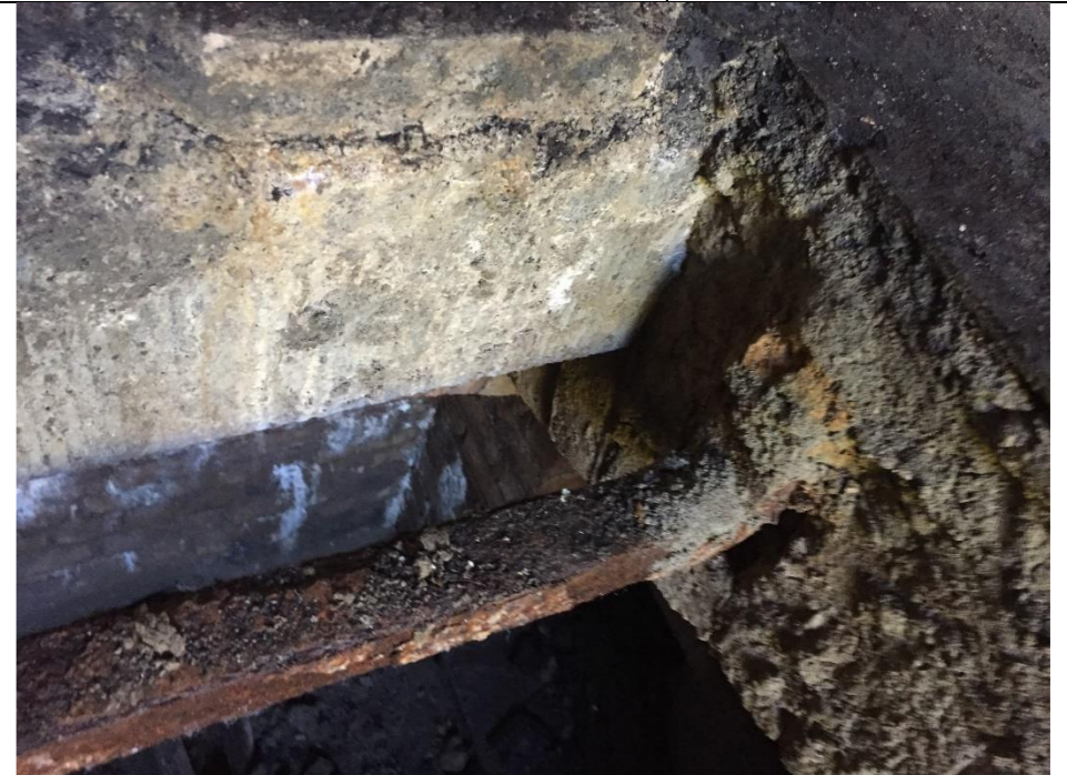
View of wrought-iron anchor straps for supporting the floor
