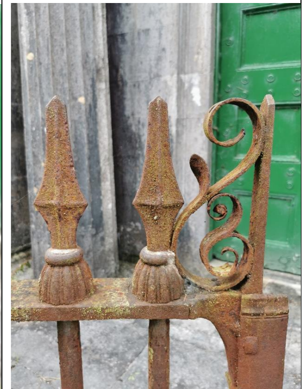
Wrought and cast-iron railing detail
