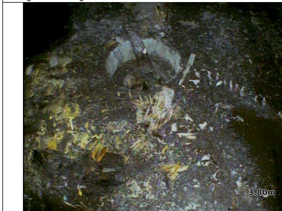
Wrought-iron fixing above central vent
