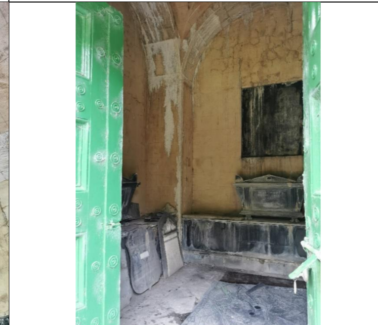
View through entrance doors to mausoleum interior
