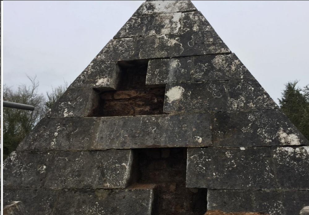
Stone blocks removed to upper pyramid during opening up works 2022
