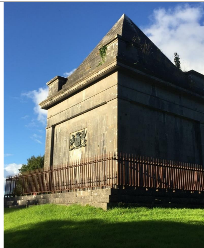
View of the mausoleum from the south
