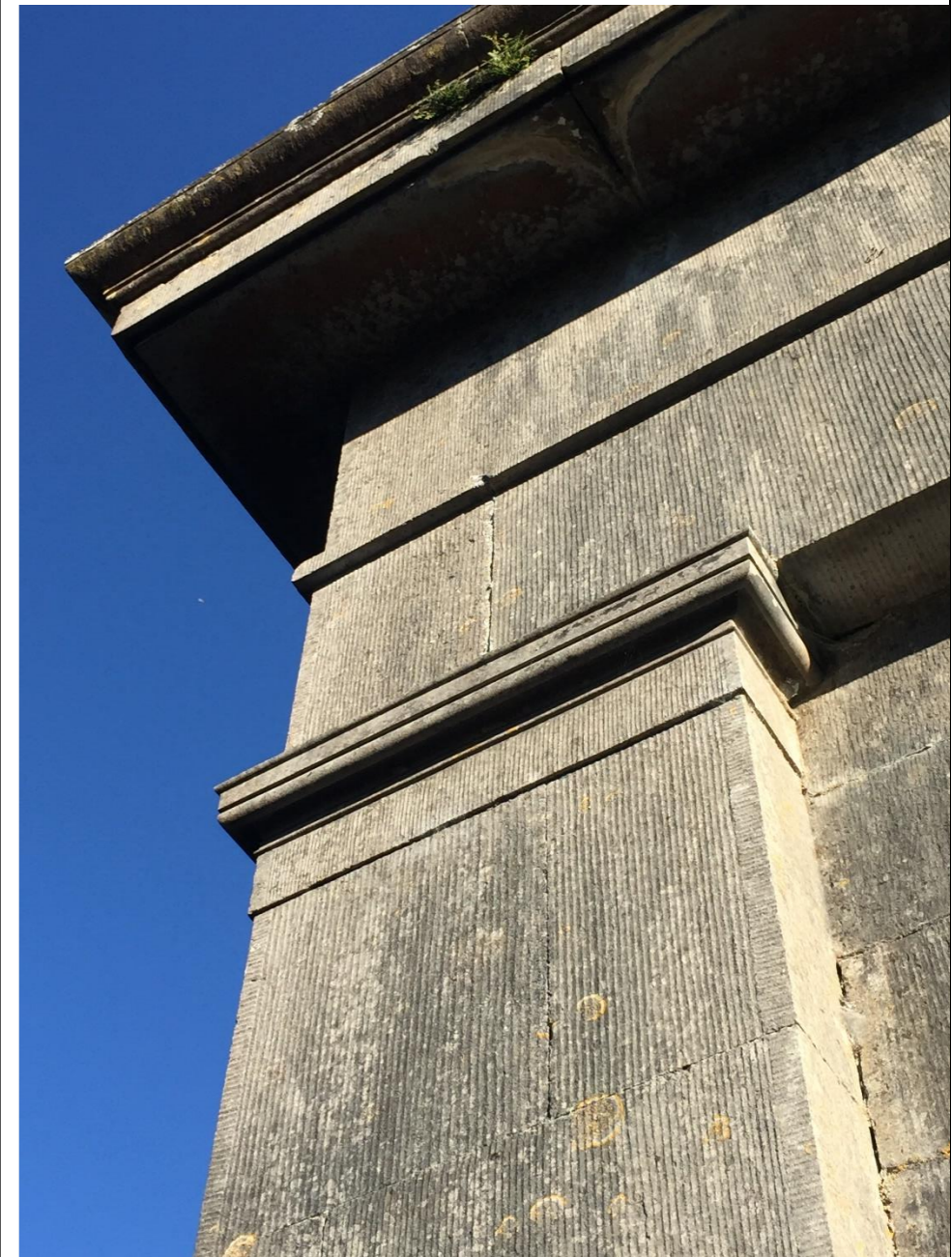
Chiselled limestone ashlar detailing
