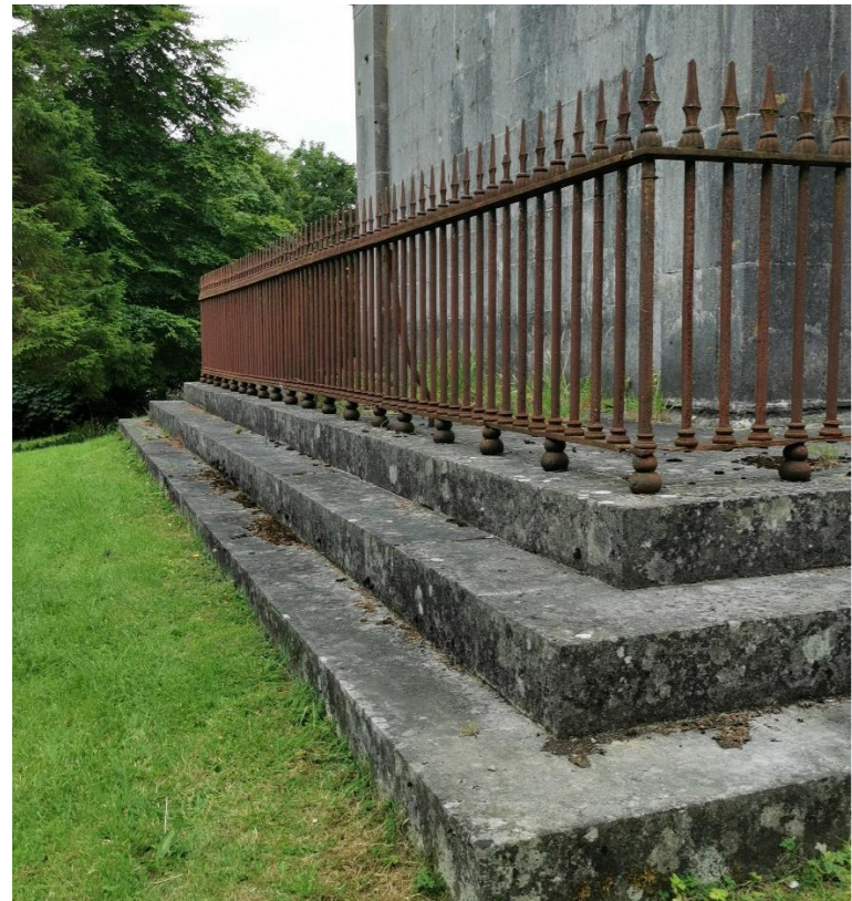
Limestone stepped threshold and railings
