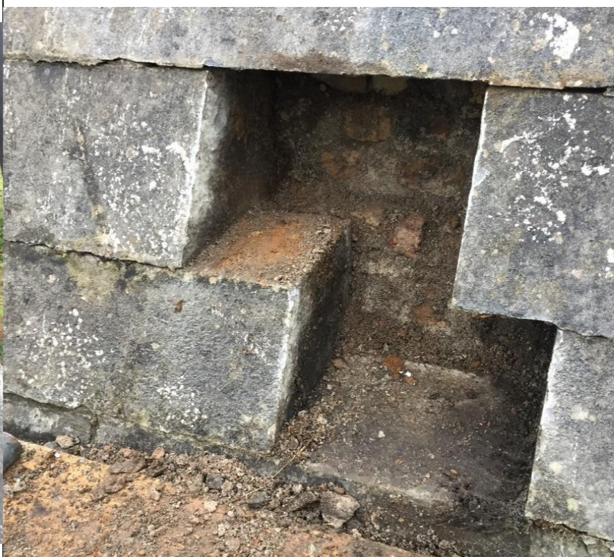
Ashlar limestone blocks removed revealing inner brick structure
