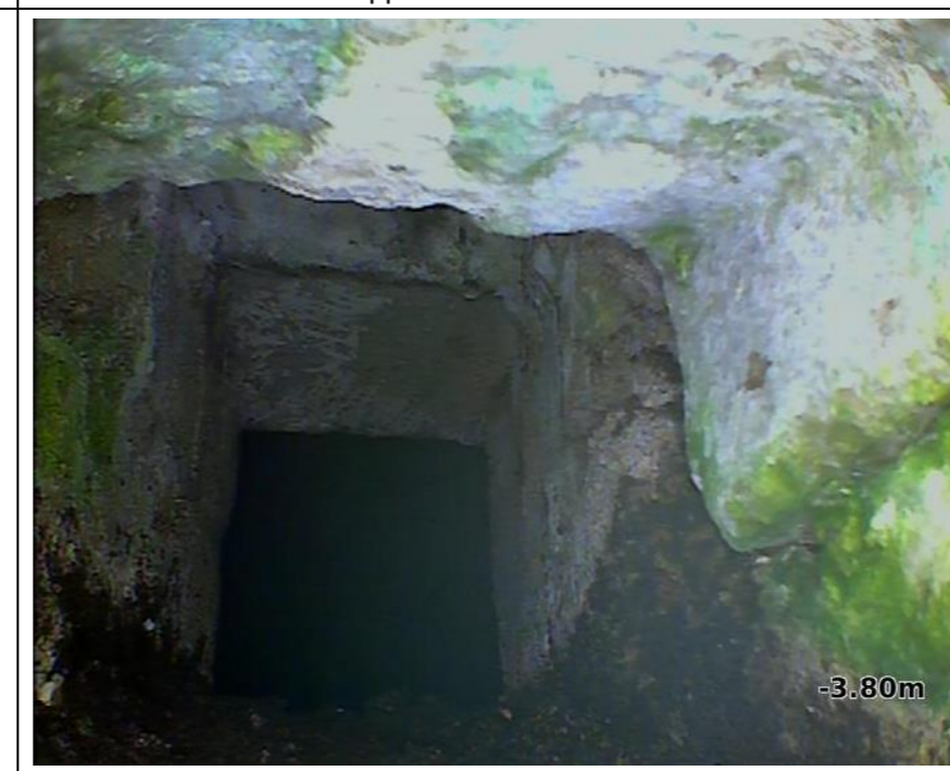
Interior view of vent opening
