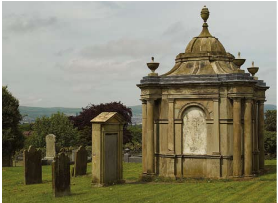
The Greg Mausoleum in the cemetery. It was probably designed by Roger Mulholland, and its brick core is rendered and detailed with cut stone. It has recently been restored
